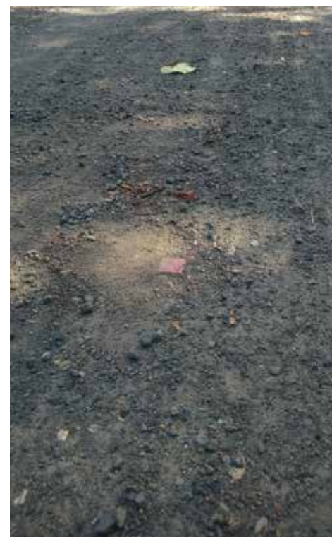
These pink caps placed every 50 feet along the trail represent the proposed centerline.
