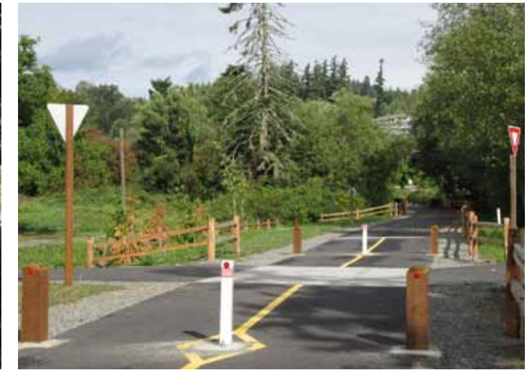
Intersection after; Issaquah segment
