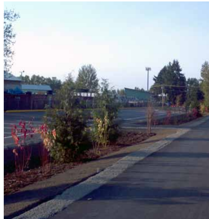
Trees are planted at least 10 feet away from the trail to promote healthy growth and prevent roots from damaging new pavement.
