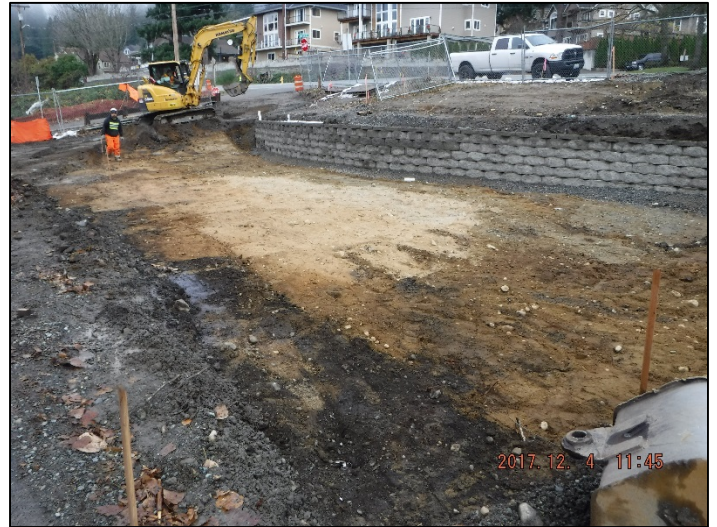
Continued earthwork at the plaza
