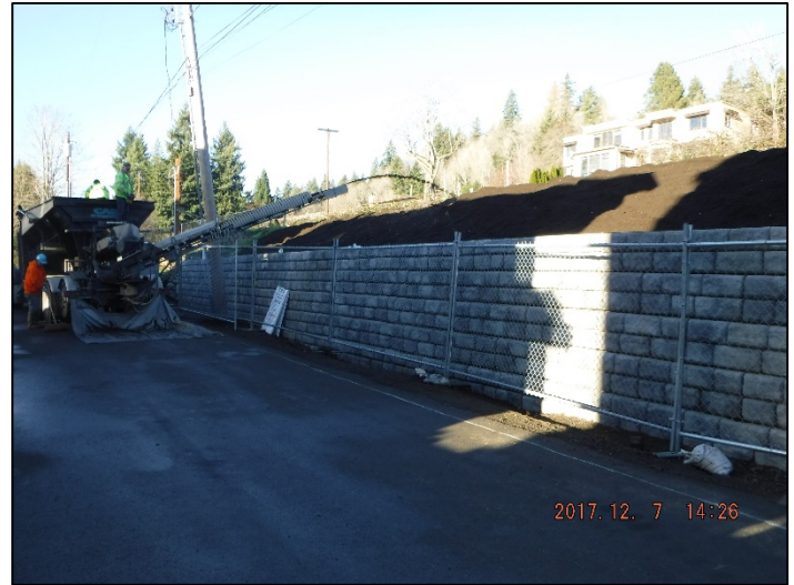
Topsoil installation above the Shorelane wall
