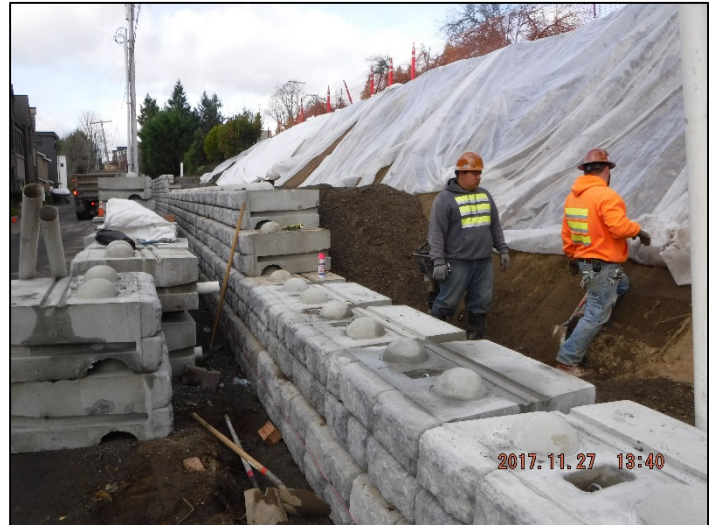
Installation of block wall at Shorelane and continued earthwork
