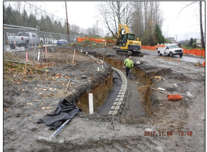
Installation of block wall at plaza and continued earthwork
