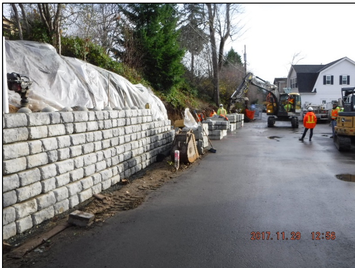
Shorelane wall block installation
