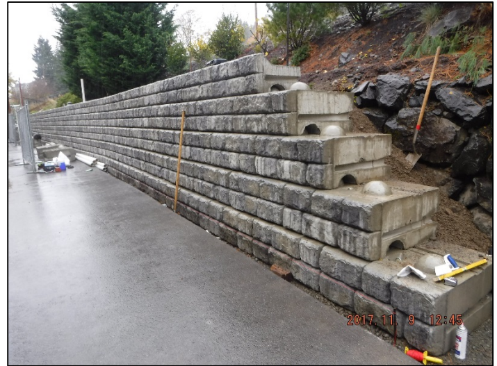
Rediwall block installation on Shore Lane
