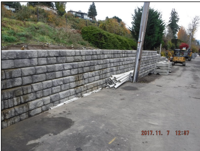
Rediwall block installation on Shore Lane
