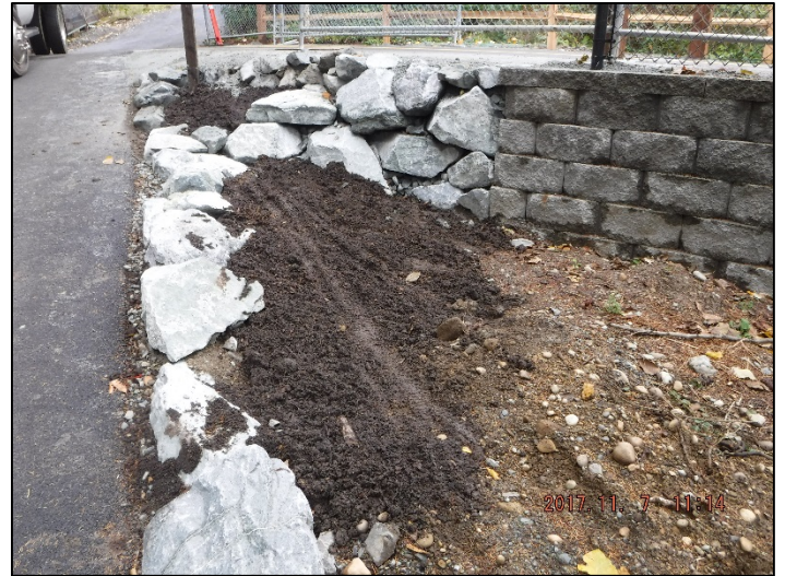
Rockery installation at Driveway 3
