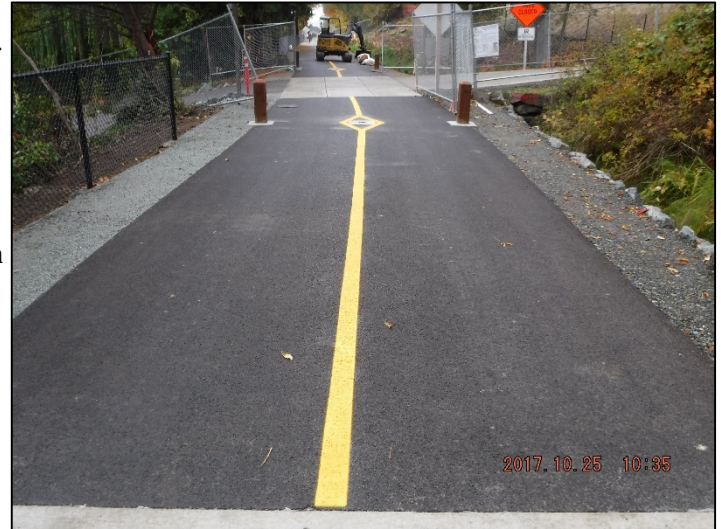
Completed project striping at Driveway 1
