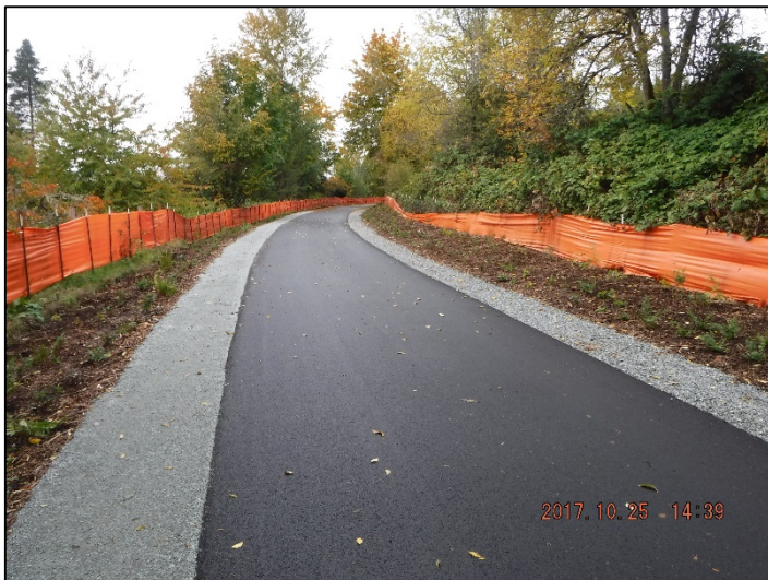
Completed planting alongside the trail between Driveway 7 and Driveway 8
