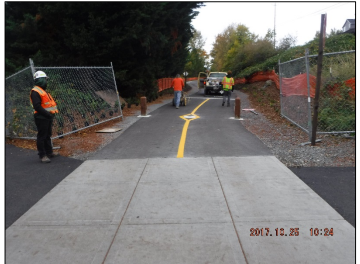
Striping installation completion at Driveway 7
