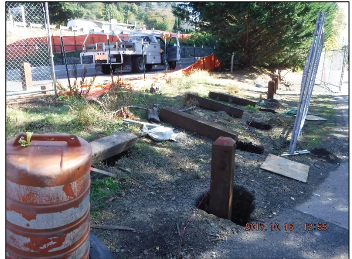
Guardrail installation at Driveway #7
