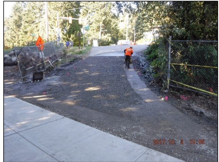
Trail asphalt grade being preparation for upcoming paving
