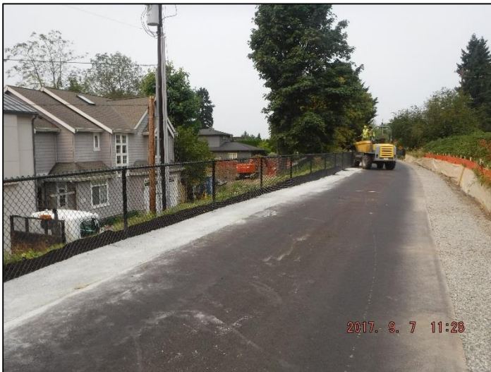
Continued installation of topsoil
