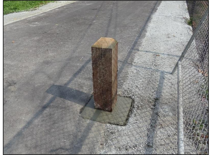
Fixed bollard installation at driveway #2
