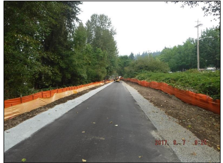
Continued installation of wood chip mulch
