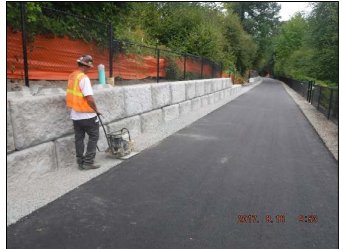
Compacting 3/4-inch ledge rock in front of Wall #8
