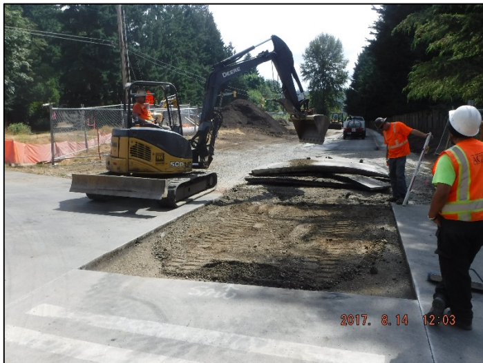
Preparing intersection at 206 th for placement of patterned concrete
