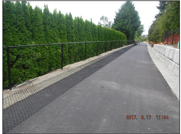
Installing chain link fence fabric, top rail and bottom rail
