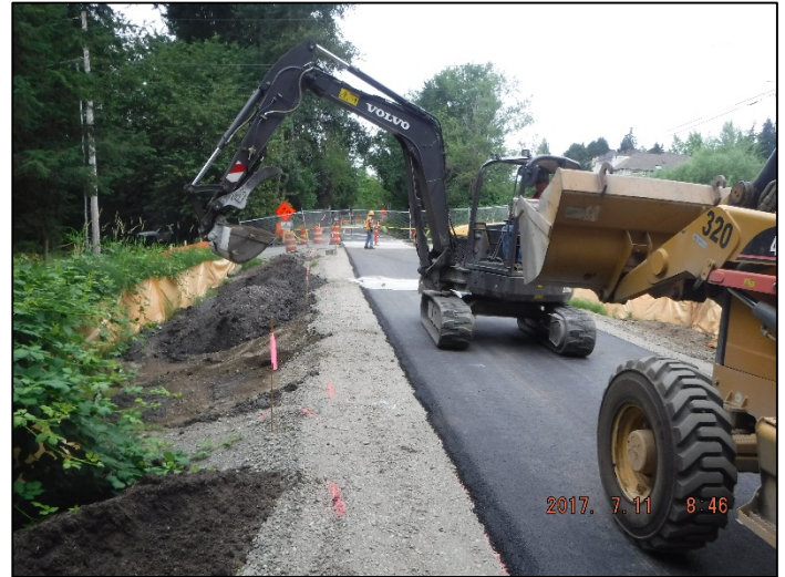
Contractor installing top soil on the slope of the trail
