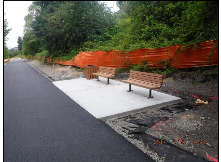
Rest area benches and garbage can enclosure installation
