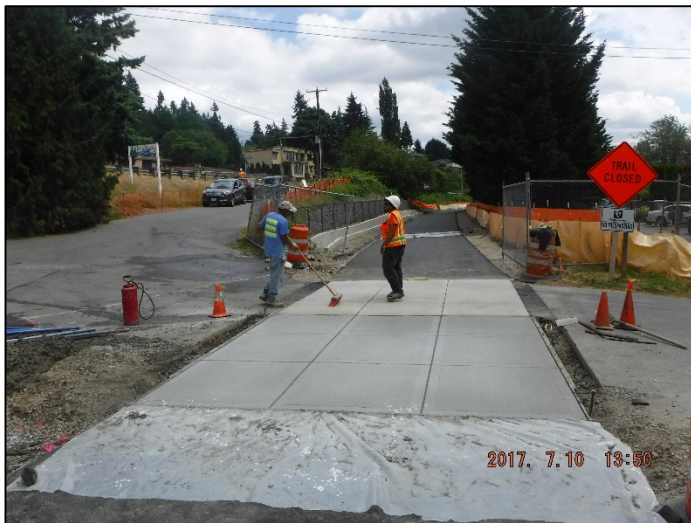
Contractor finishing a concrete intersection
