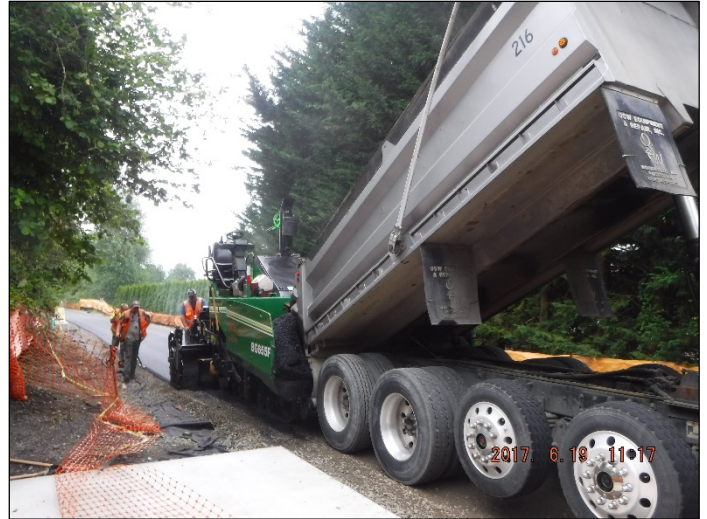
An asphalt truck depositing hot mix asphalt into the paving machine
