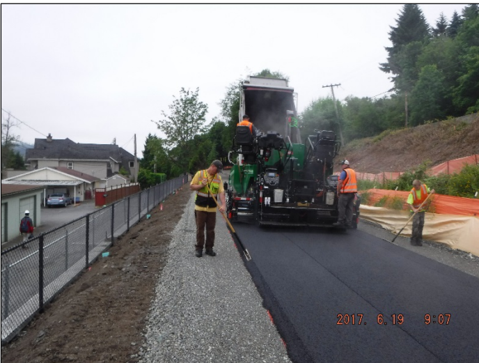
Continued installation of asphalt between driveways 2 and 3
