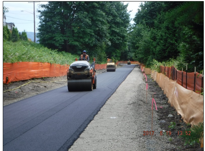
Compaction application with three double-drum vibratory rollers
