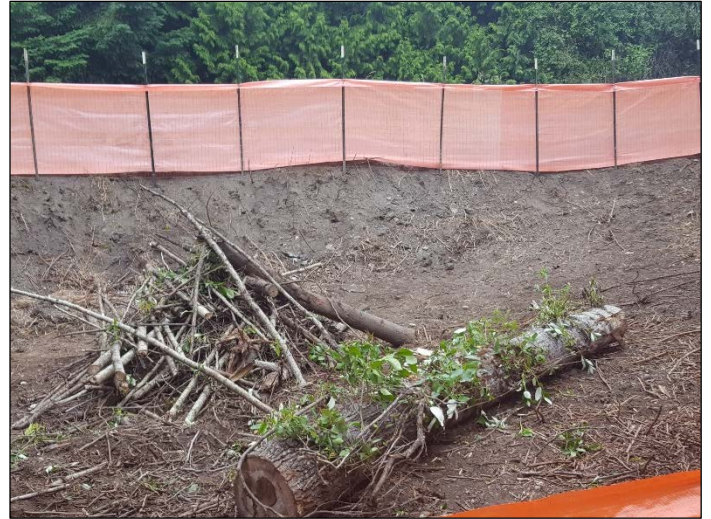
Installation of habitat logs and brush piles in the mitigation sites
