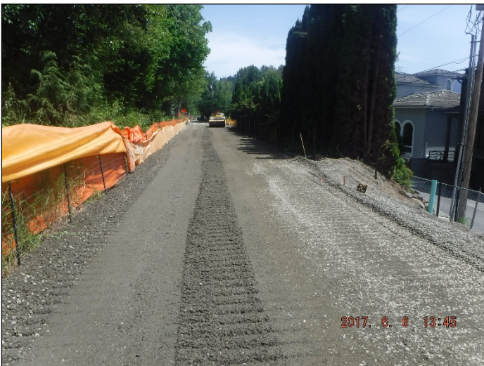
Continued fine grading of Crushed Surfacing Base Course (CSBC) for asphalt paving
