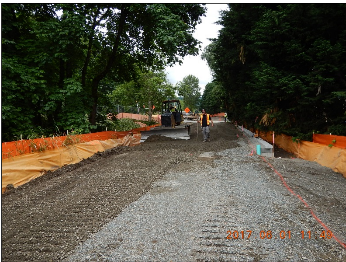
Trail grading and installation of Crushed Surfacing Base Course (CSBC)
