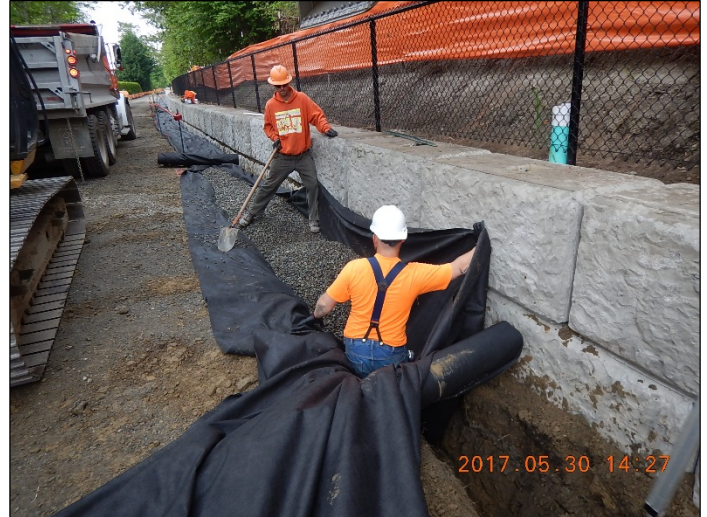
Infiltration trench installation in front of the gravity block wall 8
