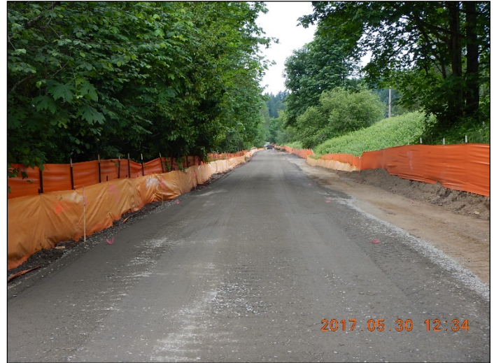
The compacted CSBC trail base in preparation for trail asphalt
