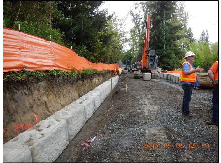
Continued installation of gravity block Wall 8.
