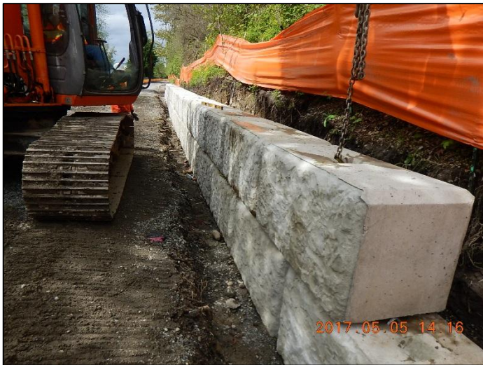
Gravity block installed at Wall #8 by the contractor.
