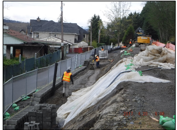
Continued installation of blocks and compaction of backfill at Wall 5
