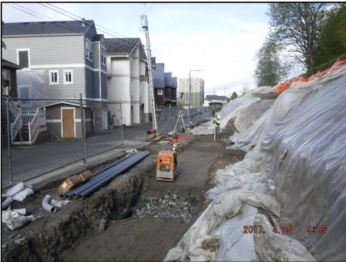
Compaction application and backfill installation for the footing of Wall 5
