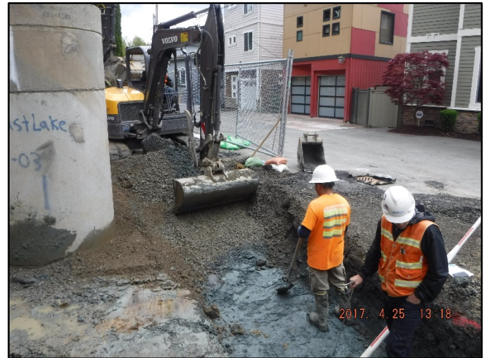
Continued excavation for Wall 3 footing near drainage structure Catch Basin 3.
