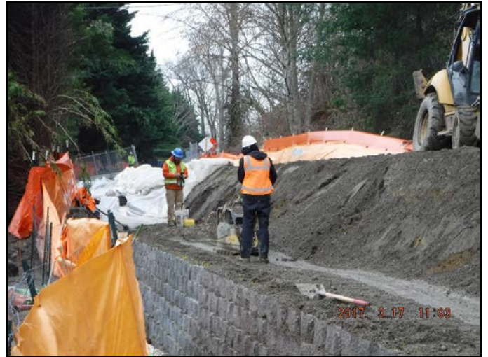
Backfill and compaction of materials behind Wall #6
