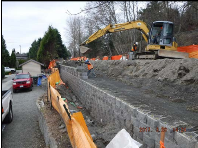
Construction of Wall #6
