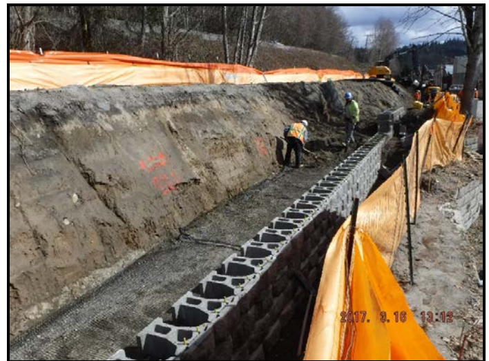
Construction of Wall #6
