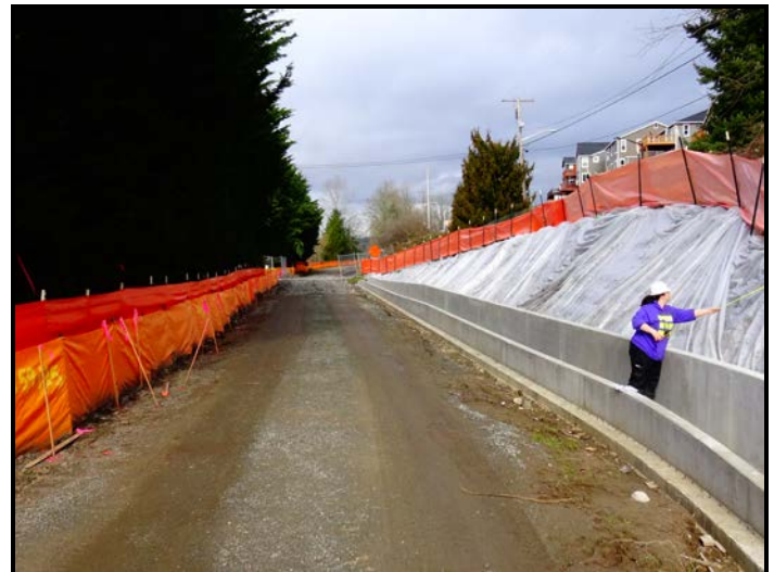
Construction of concrete channel
