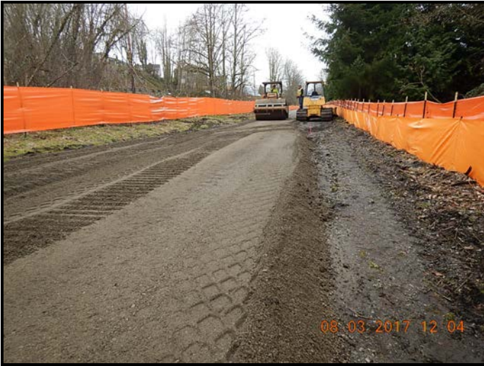
Placing CSBC material on trail
