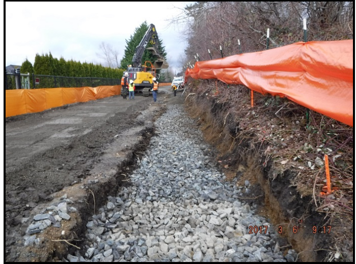
Excavating foundation for Wall #8
