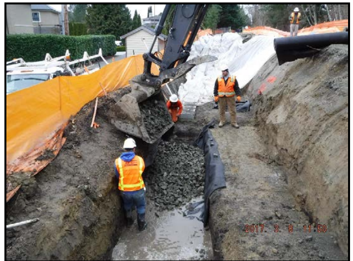
Excavation for Wall #6
