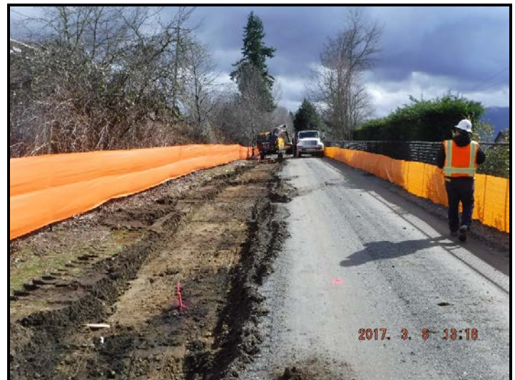
Excavating Trail Footprint
