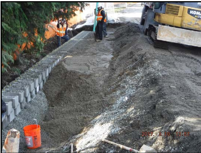
Construction of Wall #7
