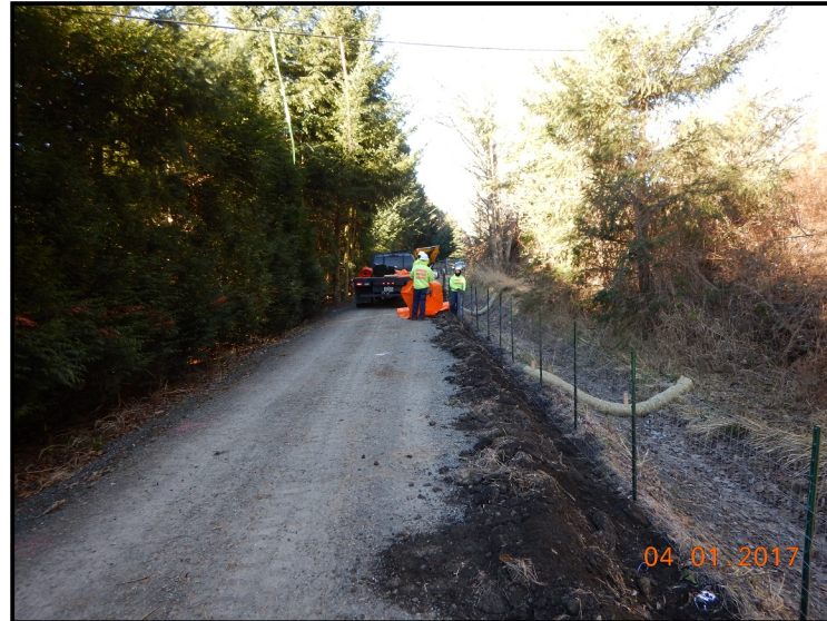
Installing erosion control fencing
