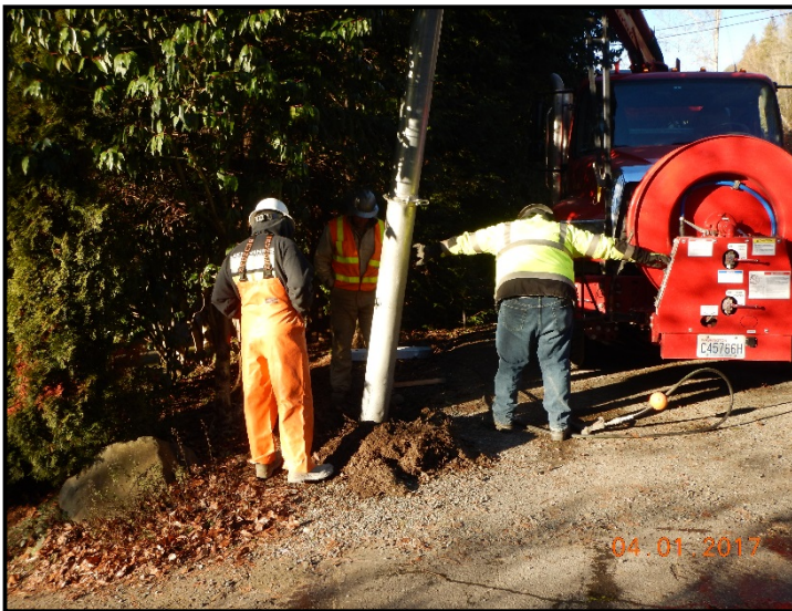
Pot holing to locate utilities
