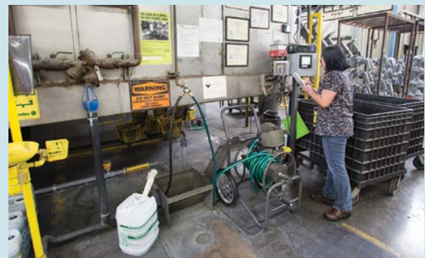
KCIW Investigator Lydia Eng checks on the instruments and backup alarms that are used to maintain water quality discharges at Precor Plant 2 Paint Shop.
