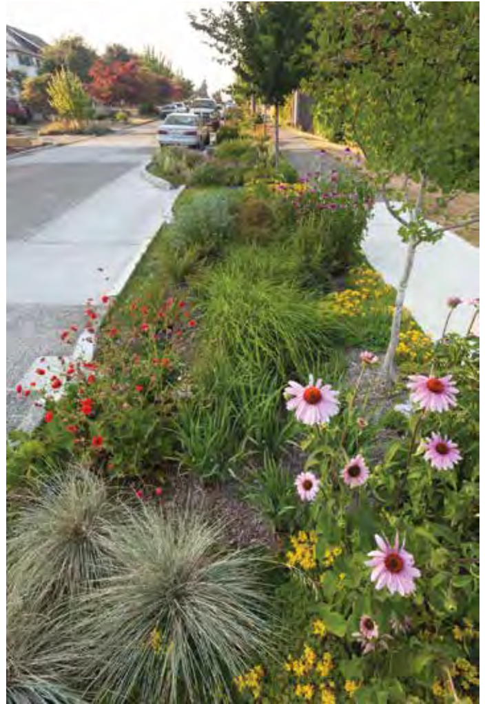
Barton Basin parking strip transformed into a roadside rain garden.
