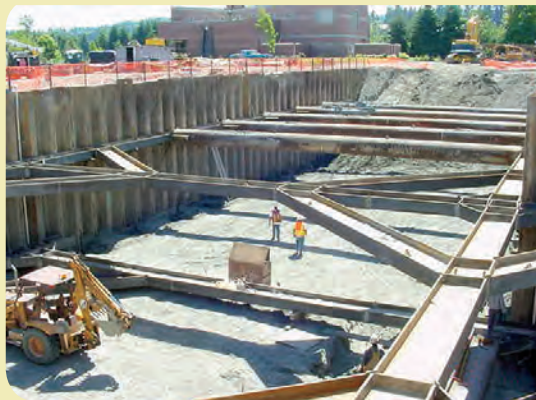
King County's six million gallon underground North Creek Storage Facility, completed in 2004, under construction.
