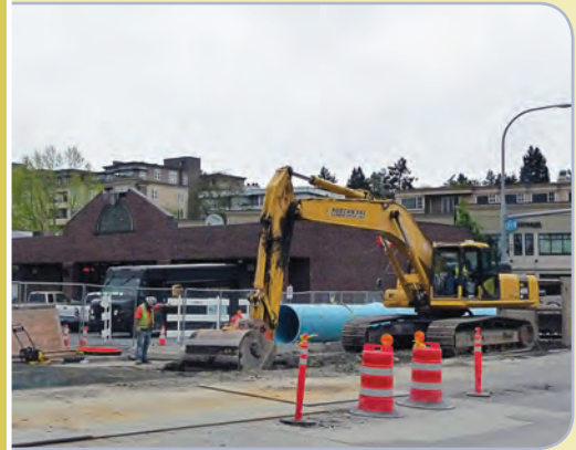
Open cut sewer pipe installation as part of a local sewer upgrade.
