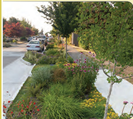
Roadside rain gardens slow, filter and absorb runoff, diverting it from the combined sewer system.
