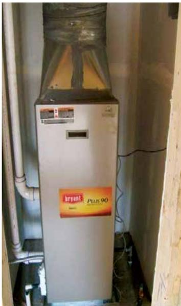
High Efficiency Energy Star Furnace with direct vent and condensate line. This furnace also includes ducted fresh air (not shown in the photo). Source: O'Brien & Company.
