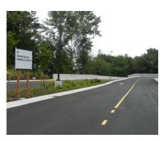
In 2012, the Solid Waste Division (SWD) used nearly 4.000 tons of **HMA** containing RAS at the new **Bow Lake** Recycling and **Transfer Station** site and nearly
