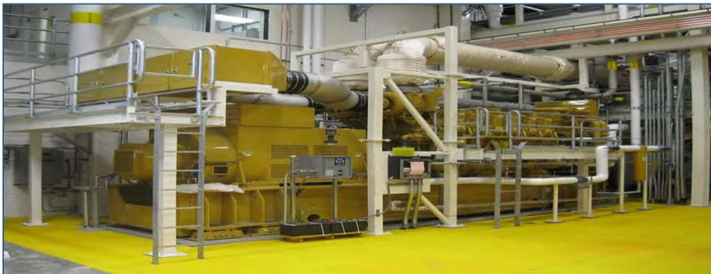
Figure 18. West Point Treatment Plant Cogeneration System
