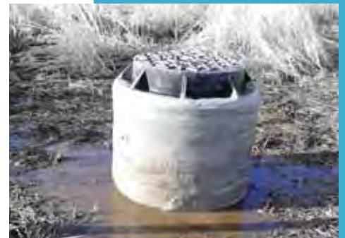
Manhole raised above water and sealed
