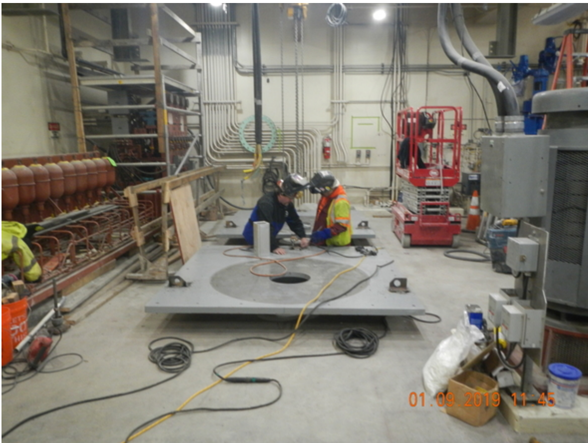
Workers inside the Sunset Pump Station.
