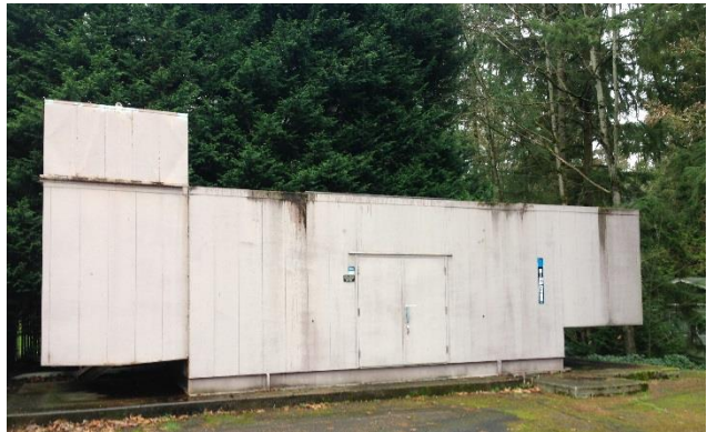
Generator enclosure at Heathfield Pump Station (shows existing color)
