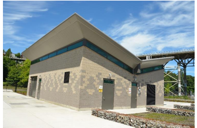
King County's contractor is working to return the Magnolia Wet Weather Facility subsurface storage tank to service, storing excess stormwater and wastewater in heavy rains.
