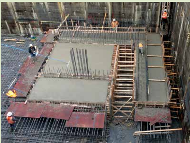
King County's contractor pours the concrete base slab of the new Rainier Valley storage tank.
