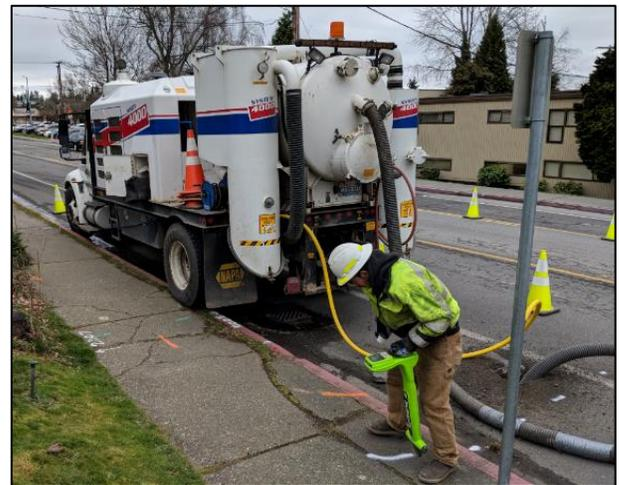
*Typical equipment used for potholing.*
