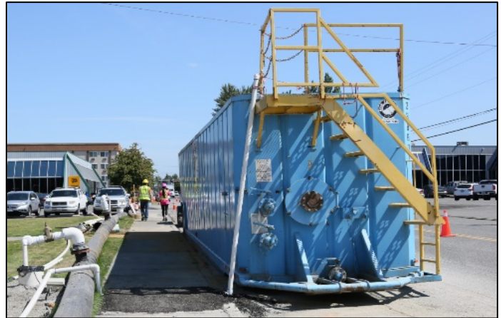
Dewatering tanks and pipes will be reinstalled.
