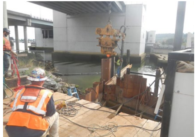
Crews begin driving sheet pile at the outfall project site.
