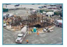
December 2018: Crews at the treatment station installed a concrete slab at the bottom of the underground Influent Pump Station. Trucks brought in concrete to pour and a platform was built to assist activities.
