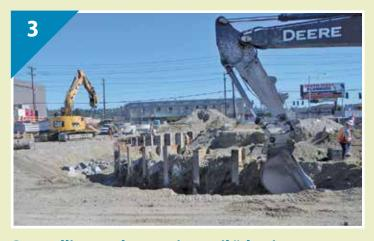
**Controlling and removing soil "shoring** and excavation": Shoring is the support system used to hold back soils during underground construction. While shoring comes in many forms, we will use trench boxes for roadway work. Once trench boxes are installed, crews will remove soil or "excavate" a trench for the work area.
