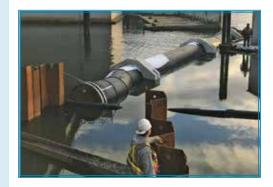
**February 2019:** A section of the outfall pipe was floated into position before the sun set and then sunk at night to take advantage of the tide.
