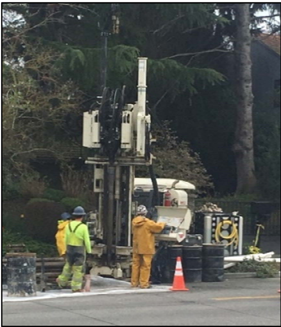
Drilling and grouting stabilized the area along the pipe under West Galer Street.
