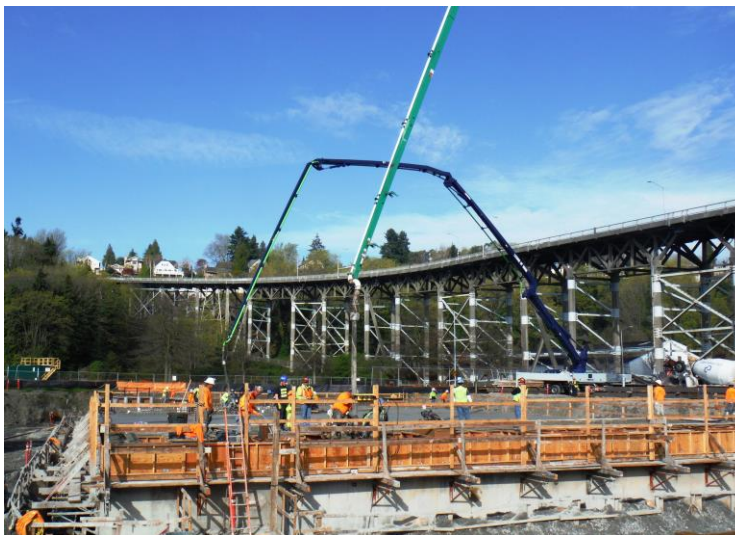
Crews installing concrete lid for storage tank
