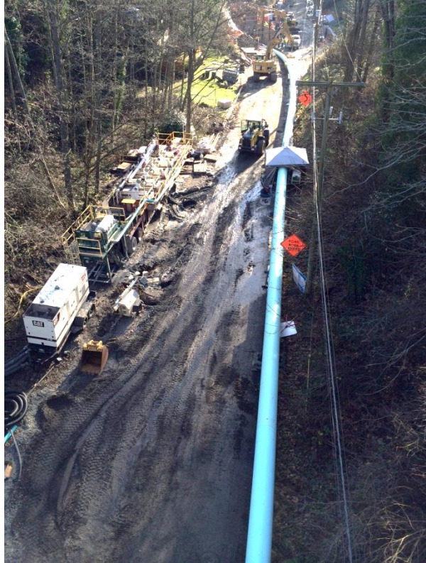
View from the West Howe Street bridge of the pipeline pullback down 32 nd Avenue West.
