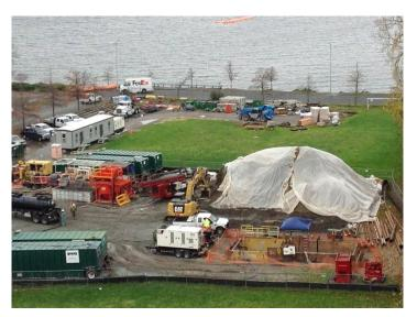
pipeline into the drilled borehole. While the pipe to be pulled back is currently laying along 32<sup>nd</sup> Avenue it will be pulled back through the borehole by equipment on the 23<sup>rd</sup> Avenue West site. The pipeline must be pulled through in one continuous effort that is expected to last for two days.
