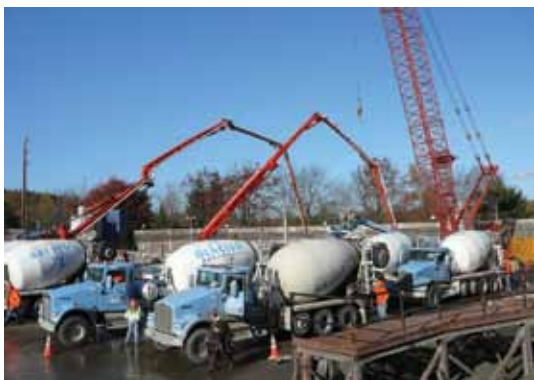
Example of concrete trucks pouring a base slab
