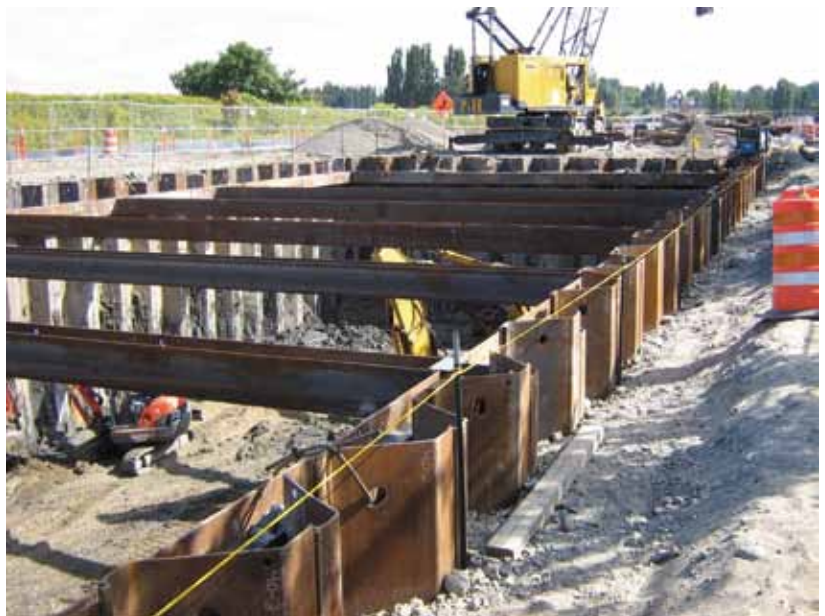
Example of excavation within the shoring system taking place
