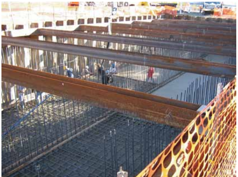
Example of installation of the base slab
