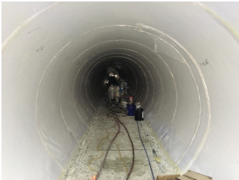
The pipe interior after it has been lined with the protective material.
