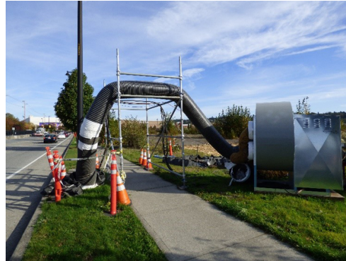
Odor control and ventilation along the pipe length ensure the conditions in the pipe are safe for crews to work inside.
