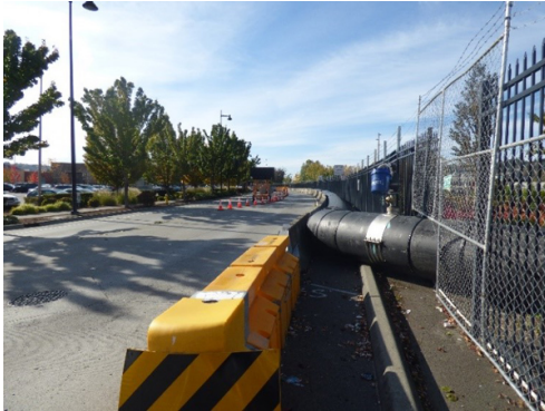
The bypass pipe is installed along a road. A concrete border and cones are used to guide traffic while work is underway.
