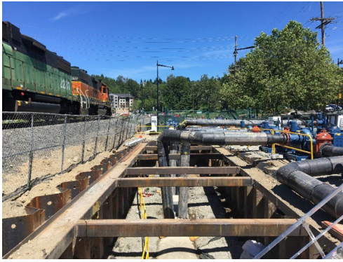
The excavated intake pit allows crews to prepare for diverting water from the pipe in preparation for pipe lining.
