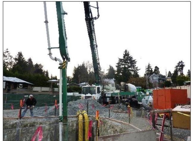
*A pump mounted on a truck pours concrete deep in the excavated area to form the base of the CSO tank.*
