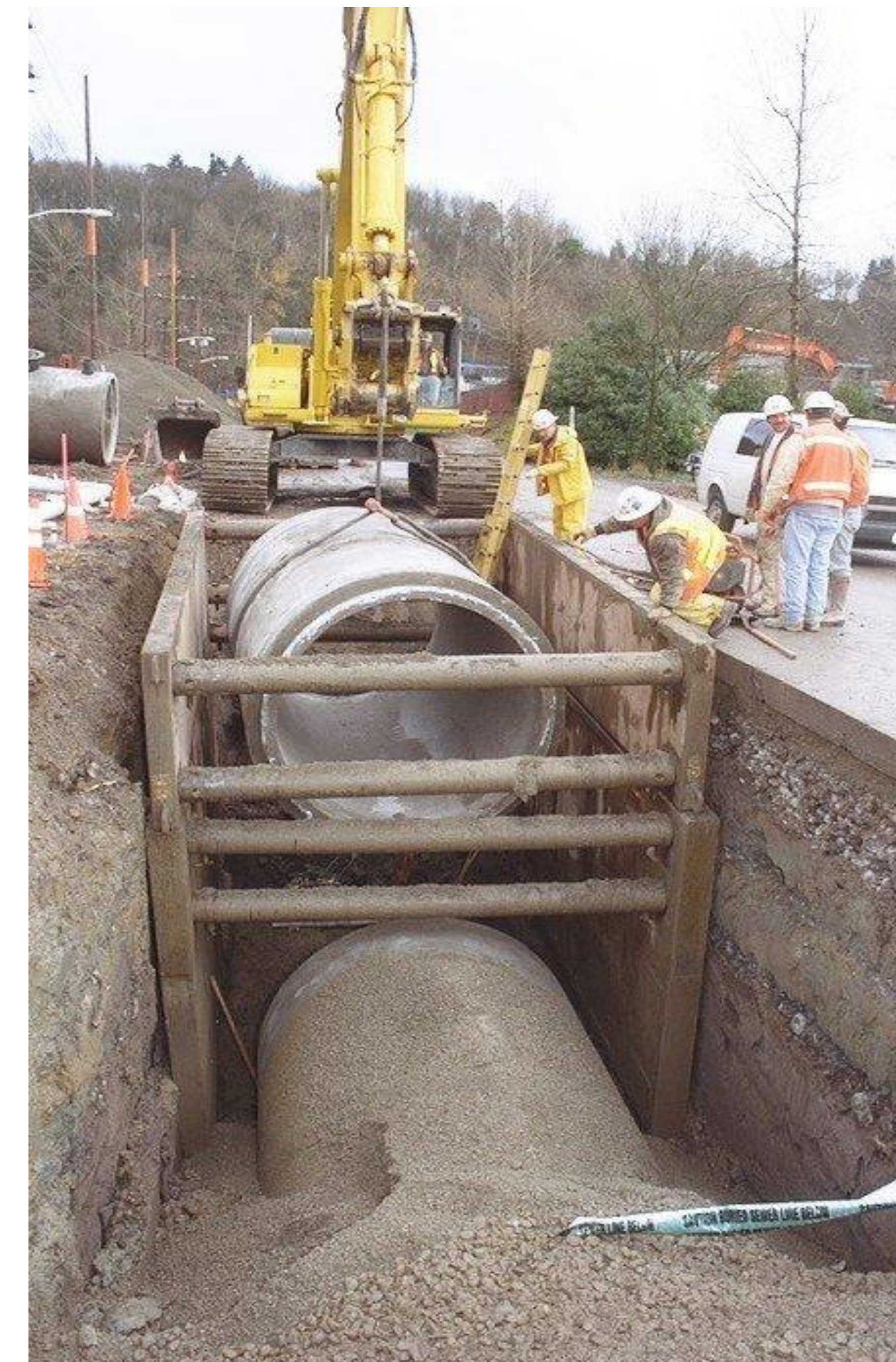
Connecting storage tank to pump station
