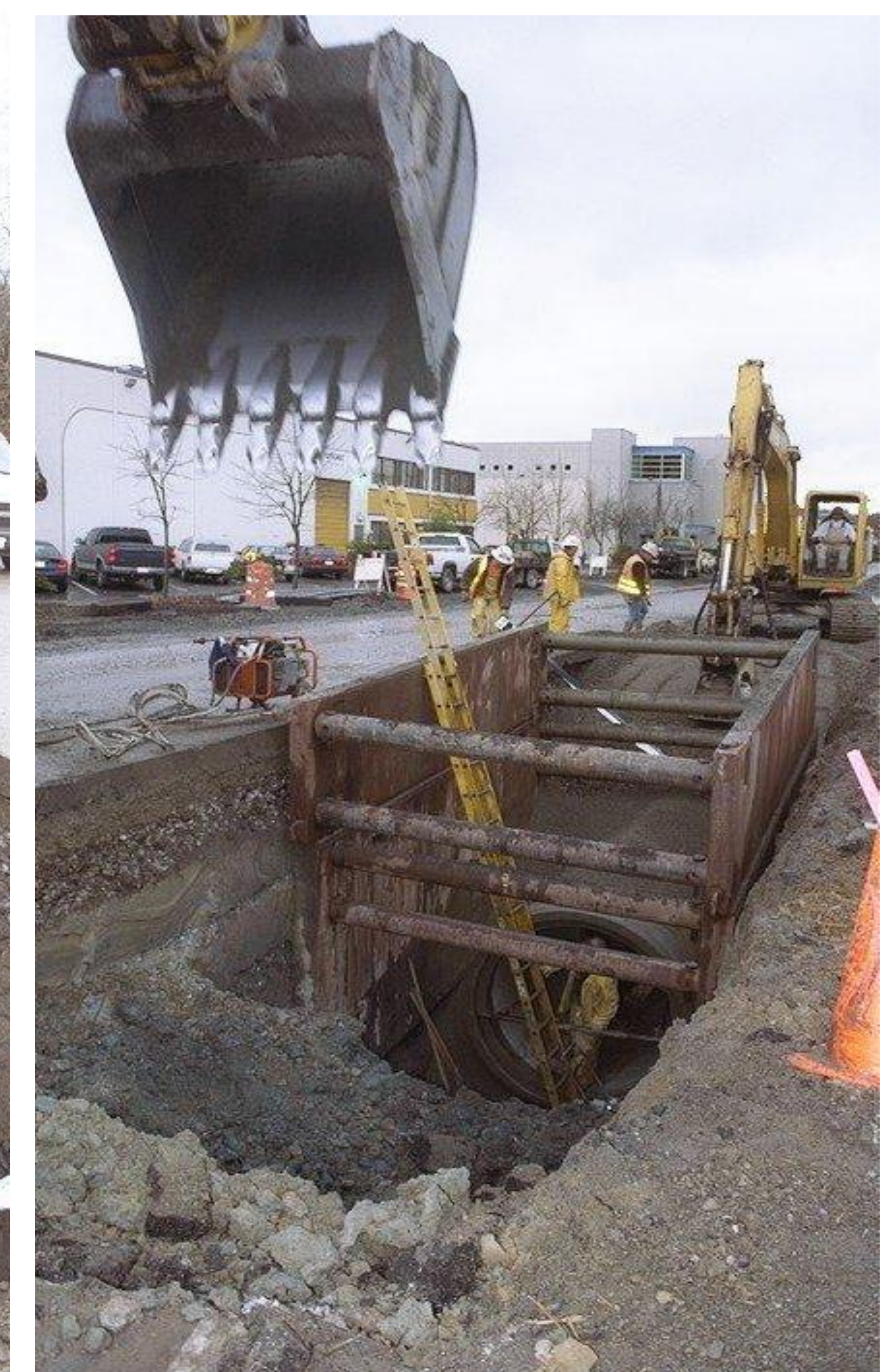
Connecting storage tank to pump station
