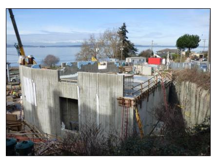
Crews are now conducting mechanical and electrical work inside the facility and have started to backfill soil behind the building.
