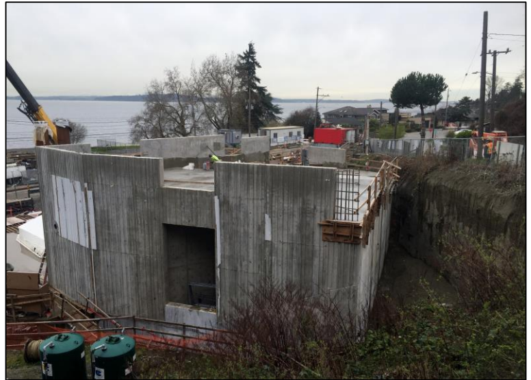
Backfilling behind the facility building is underway to cover the soil nail wall.
