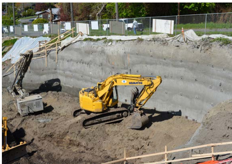
The soil nail wall will stabilize the site's hillside during construction of the control facility.
