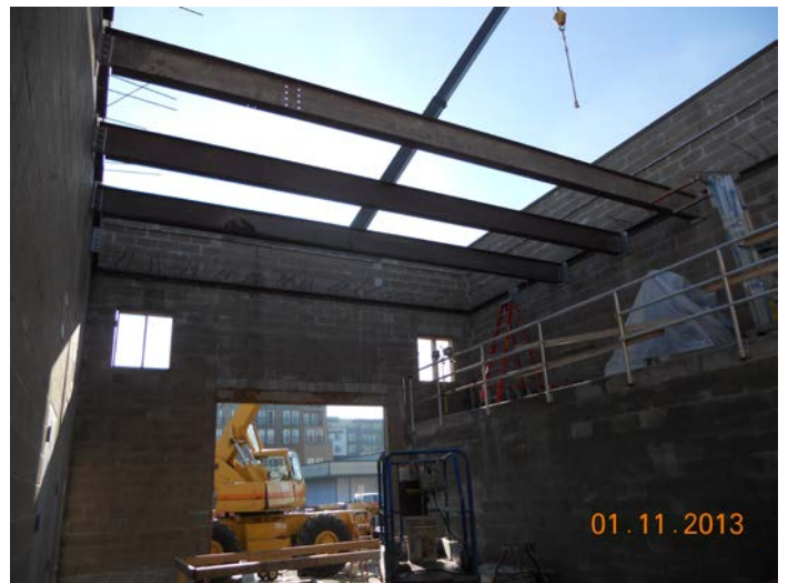
Pump station exterior wall construction.
