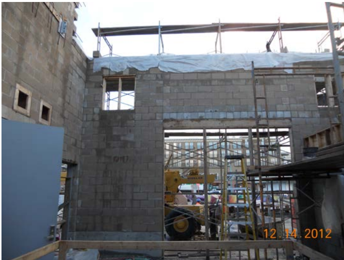
Pump station exterior wall construction.
