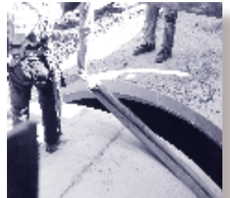
A secondary suspension system is used to fit the pipe segments together.
