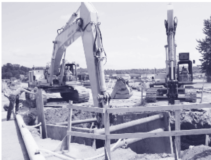
Trenching to install a new sewer.
