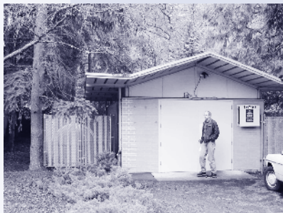
Existing Hidden Lake Pump Station
