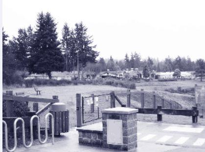
New sewer through park
