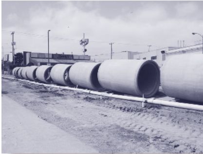
A trenching project in progress.
